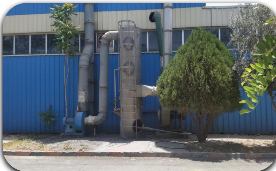
Air Washer System Installation at Saba Battery
