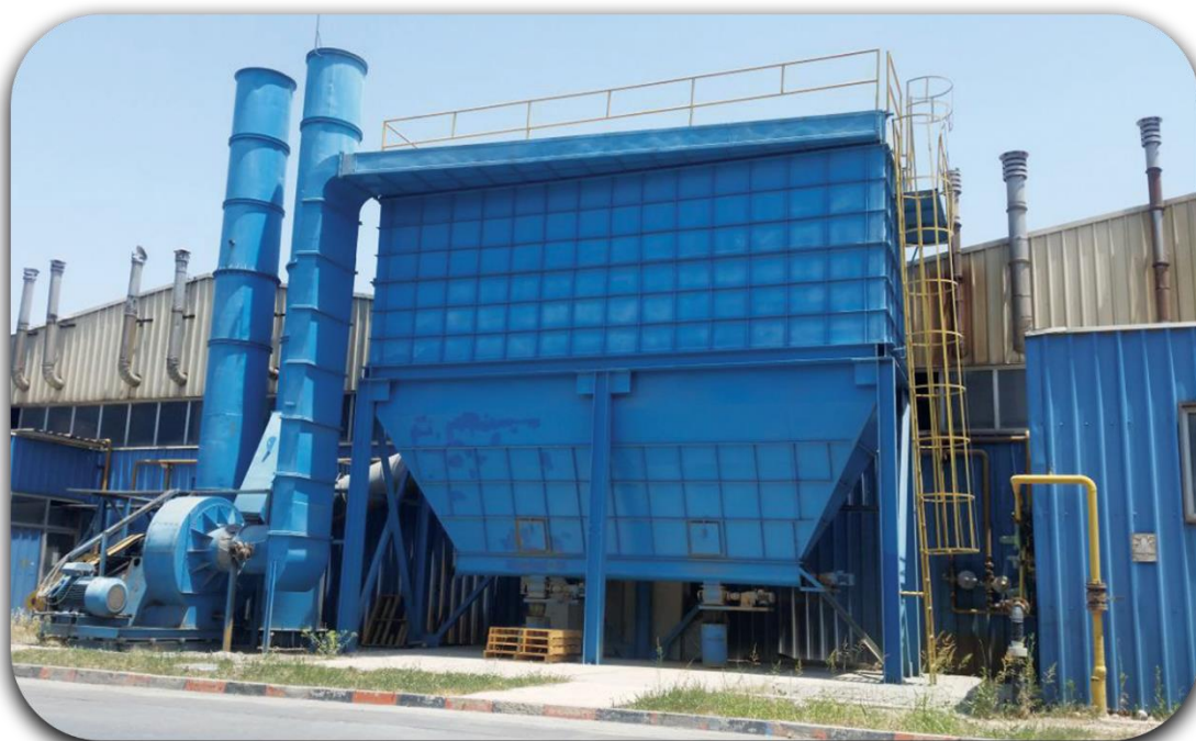
Construction and Installation of Bag Filter for Saba Battery
