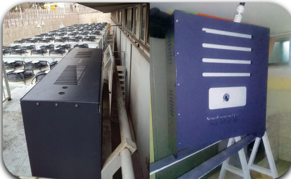
Construction and Installation of a 400-gram Ozone Generator for Tehran Heart Hospital
